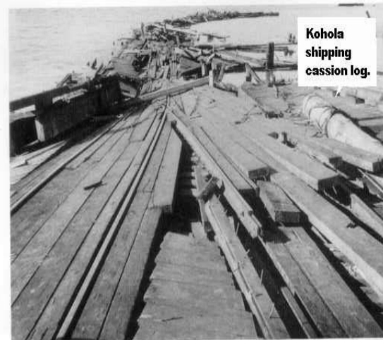
View of wrecked pier. Submerged Stern of Quinalt Victory is at upper right. (U.S. Navy)
